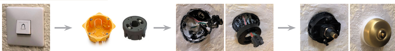
Attach the Garby box inside the existing box.
